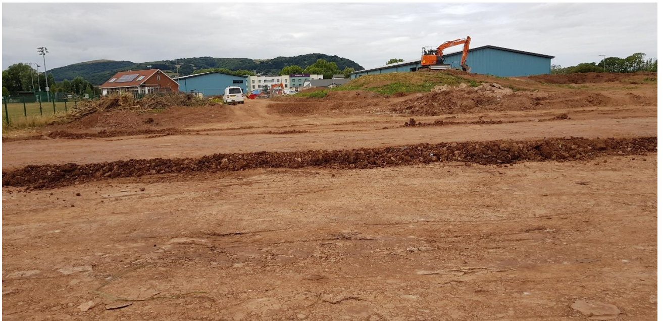
Raising the level of the site with spoil from the industrial land.
